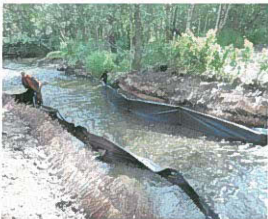
The WSWCD Crew repairing stream banks on Wasilla Creek
