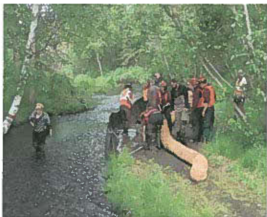
The WSWCD Crew placing Coir log For the Little Meadow Creek Project.
