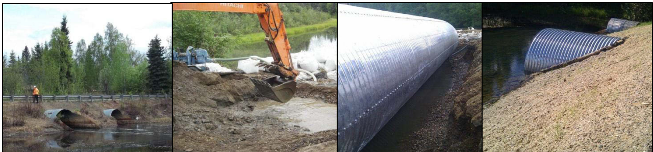
Persinger culvert was replaced during 2012. The new culvert will improve fish passage and benefit other wildlife.
