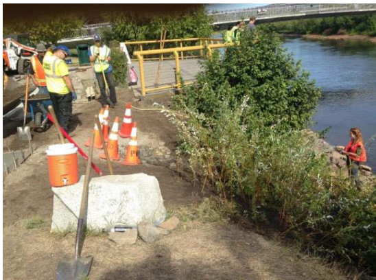
Shoreway park restoration, before (above) and after the concrete was removed and willows planted (right)
